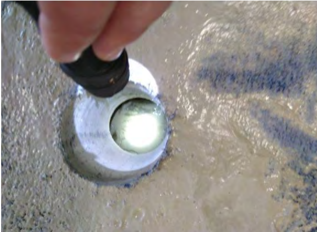
Photo 3: BH114 showing the void beneath the concrete slab
